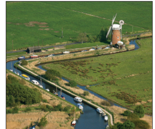
Horsey Mill (NT) used to drain the marshes but an electric pump in the shed at the side does the job now.
